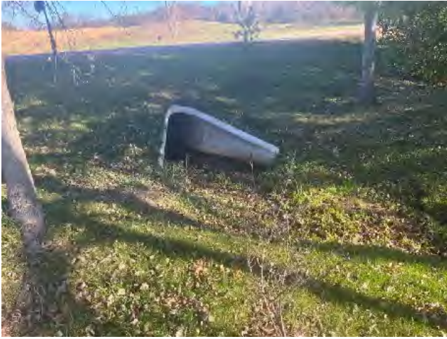
County Rd 47 Culvert
