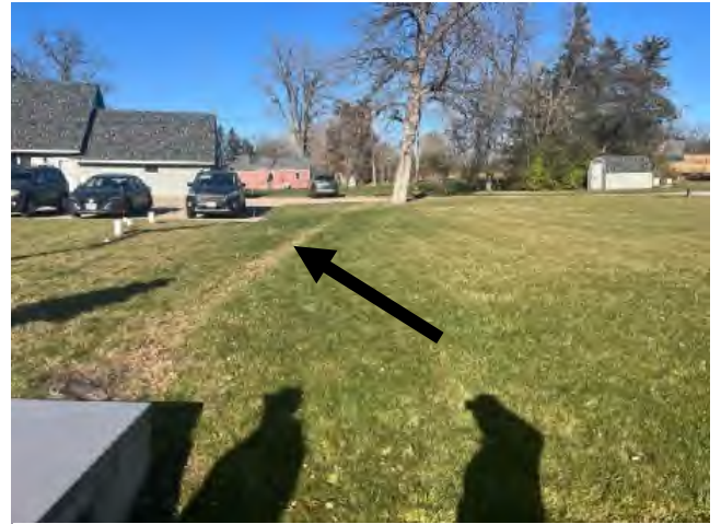
Arrow showing underground pipe/tile which is connected to driveway culvert
