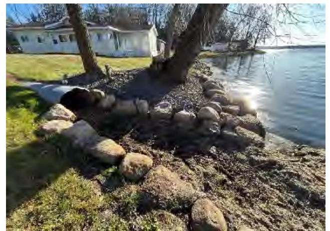
Outlet of existing drainage system
