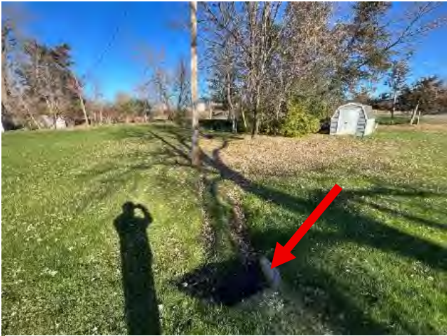
Driveway culvert receiving water from County Rd 47 culvert & runoff from property
